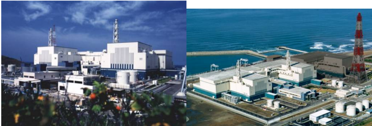
FIG. 12.1. Kashiwazaki-Kariwa Nuclear Power Station Unit 6&7 (Tokyo Electric Power Co.) (Right Photo: from left, Unit 7, Unit 6 (ABWR, 1356MWe) and Unit 5 (BWR-5, 1100MWe))
