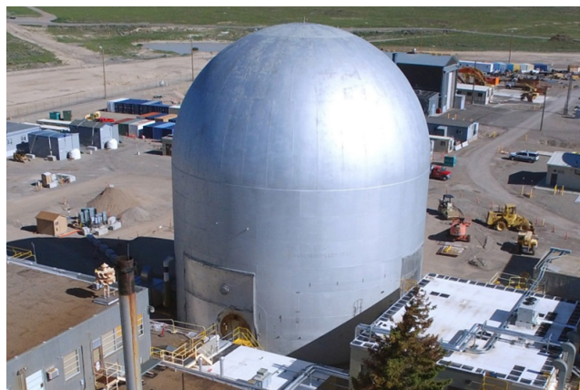
Figure 5. Exterior view of EBR-II containment, the key structure composing the DOME facility.
