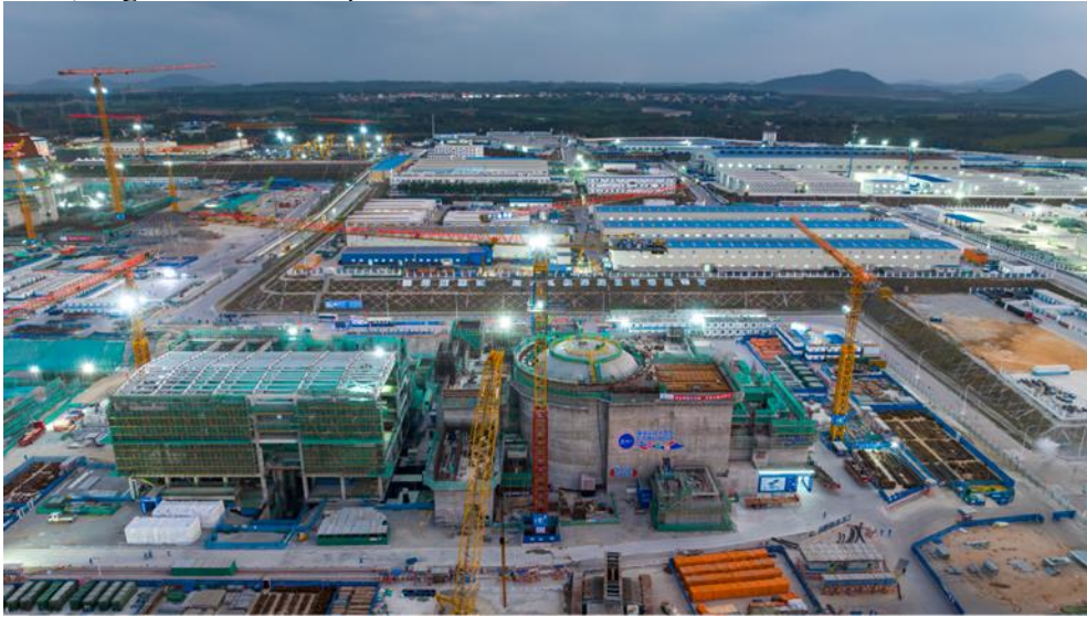
Site construction drawing in 2024
