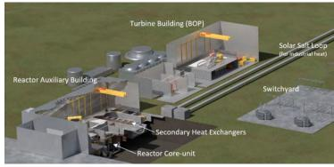
been de-fuelled to the spent fuel salt storage tanks. The de-fuelled core-unit is then moved with an overhead crane from its operating silo to a long-term storage silo inside the reactor auxiliary building. A third core-unit can then subsequently be installed in the now empty operating silo, ready to begin another 7-year operating cycle once the second operating core-unit unit reaches end-of-life and is shut down.
